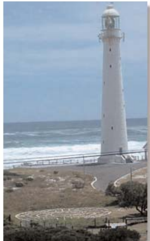
Permanent Reconciliation Labyrinth at the base of famous lighthouse landmark in Kommetjie, South Africa
